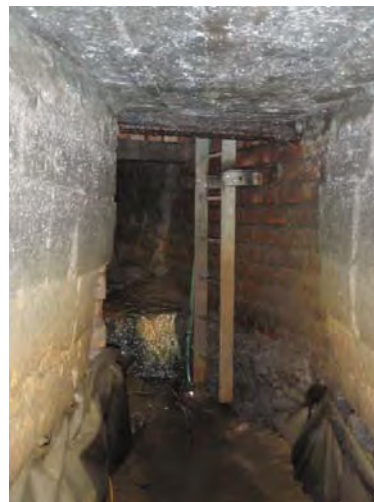
Photos of interior of Drain
