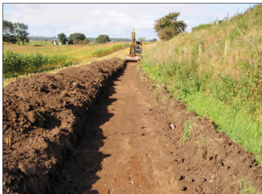
Plate 7: C16 - Evaluation trench in progress taken from East.
